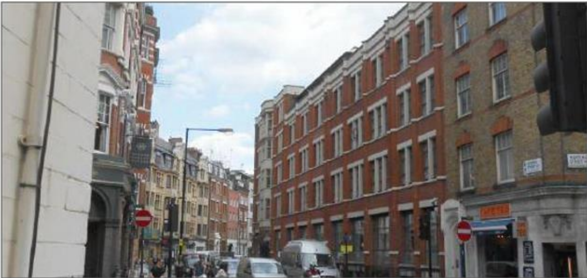
View from Cleveland Street
