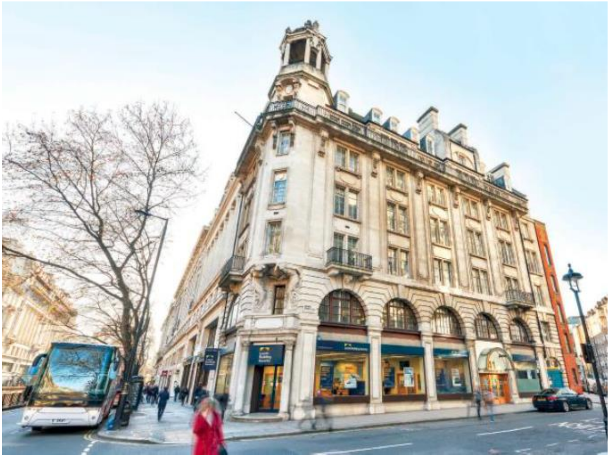
View from Kingsway
